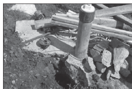
Figure 1. The slab around this capped well must be repaired to keep water from entering the well bore hole.
