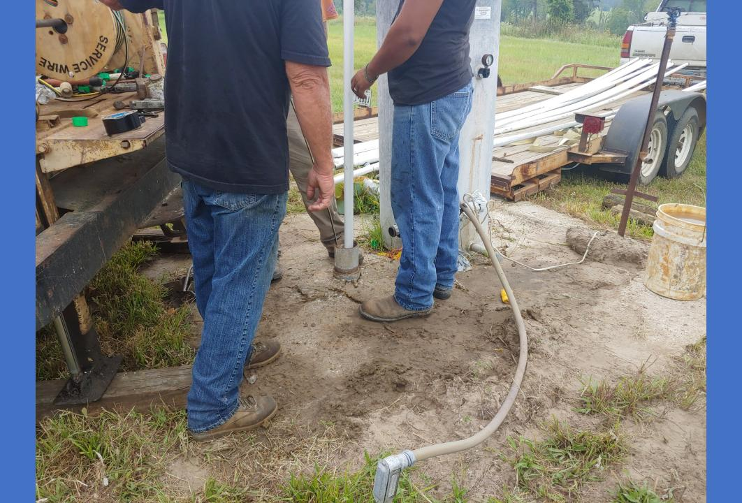
Simply lowering the pump to a new depth can normally take place in a few hours.
