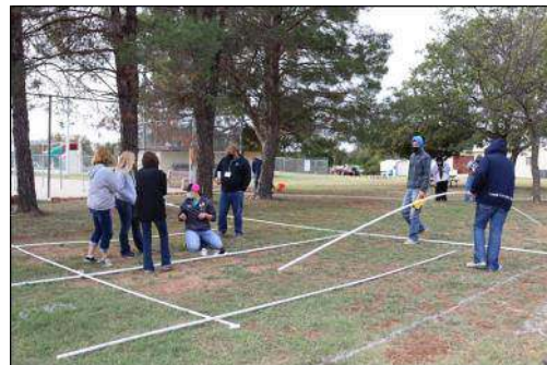
Installing lateral pipe for each station
