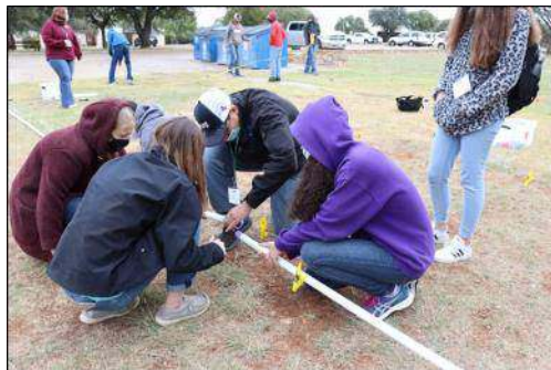
Installing the irrigation mainline
