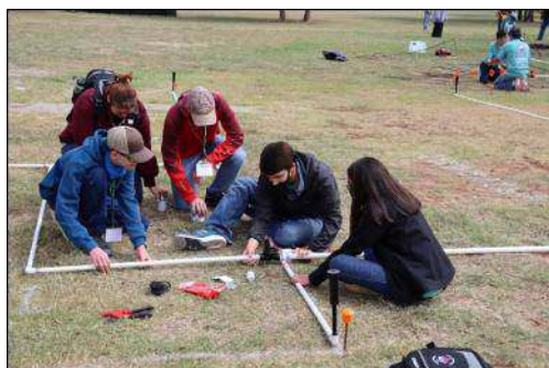
Installing control valves and sprinklers
