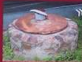
J.D. Giddings' first cistern, built in the early 1860's, is still visible today at the Giddings William House Museum. Downspouts and pipes brought water from the reservoir roof into the cistern.
