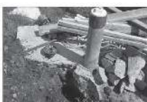
Figure 8. The abb around this cap must be packed to keep water from entering the well bore hole.
