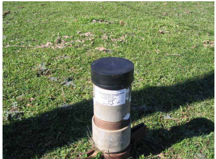
A properly capped well is one that is closed or capped with a covering capable of preventing surface pollutants from entering the well and that can sustain a weight of 400 pounds, and is constructed in such a way that it cannot be easily removed by hand.
